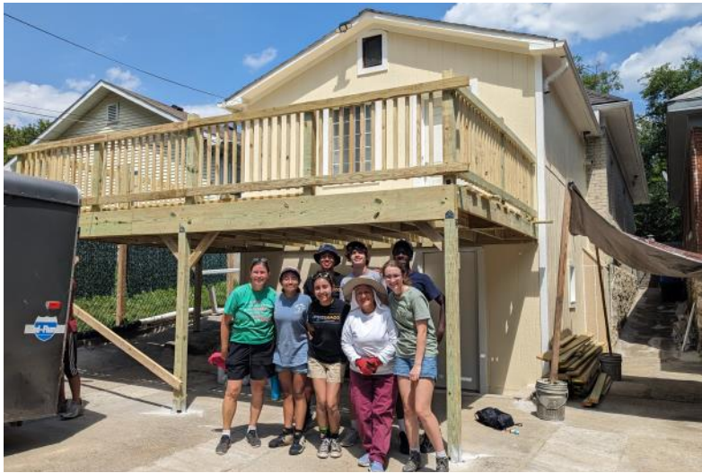
Building a Deck With Our Resident
