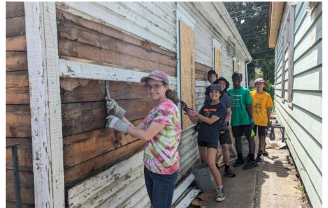
Removing Siding From a House
